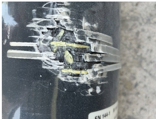
Exemplary damage of level 3 caused by structural shell fiber delamination
