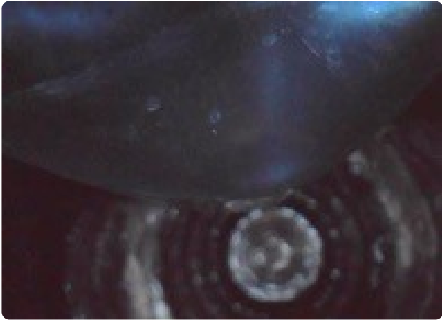
Bulging effect visible inside the cylinder
