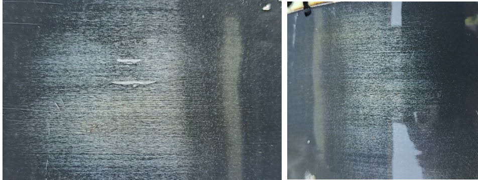
Exemplary damage of level 1 caused by high temperature or fire
